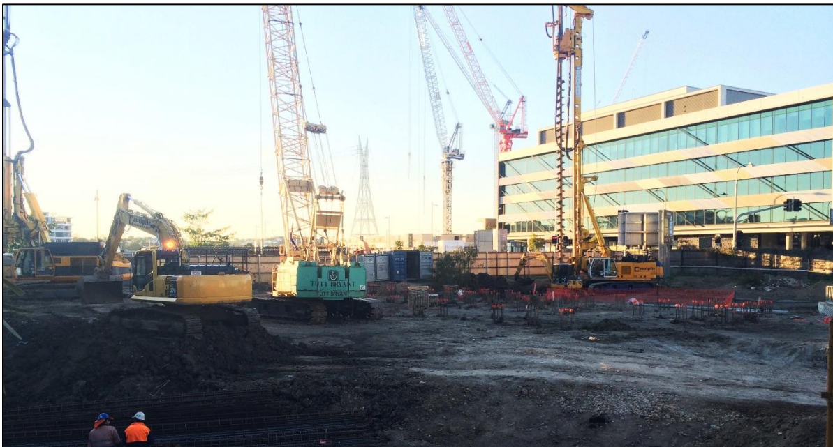
Haven Site: Complete piles with steel reinforcing awaiting pile caps.
