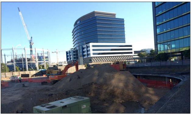
Haven Site: Pile of imported fill used to establish platforms for piling rigs. The material is now in the process of being removed from site.
