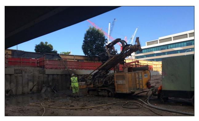
Haven Site: Drill rig establishing rock anchors for the retaining wall. The anchors are inserted on a 45 degree angle.
