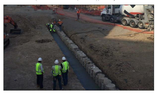
Haven Site: Secant retailing wall with the piling cap having just been poured. The tops will be trimmed off when the fresh concrete has cured.
