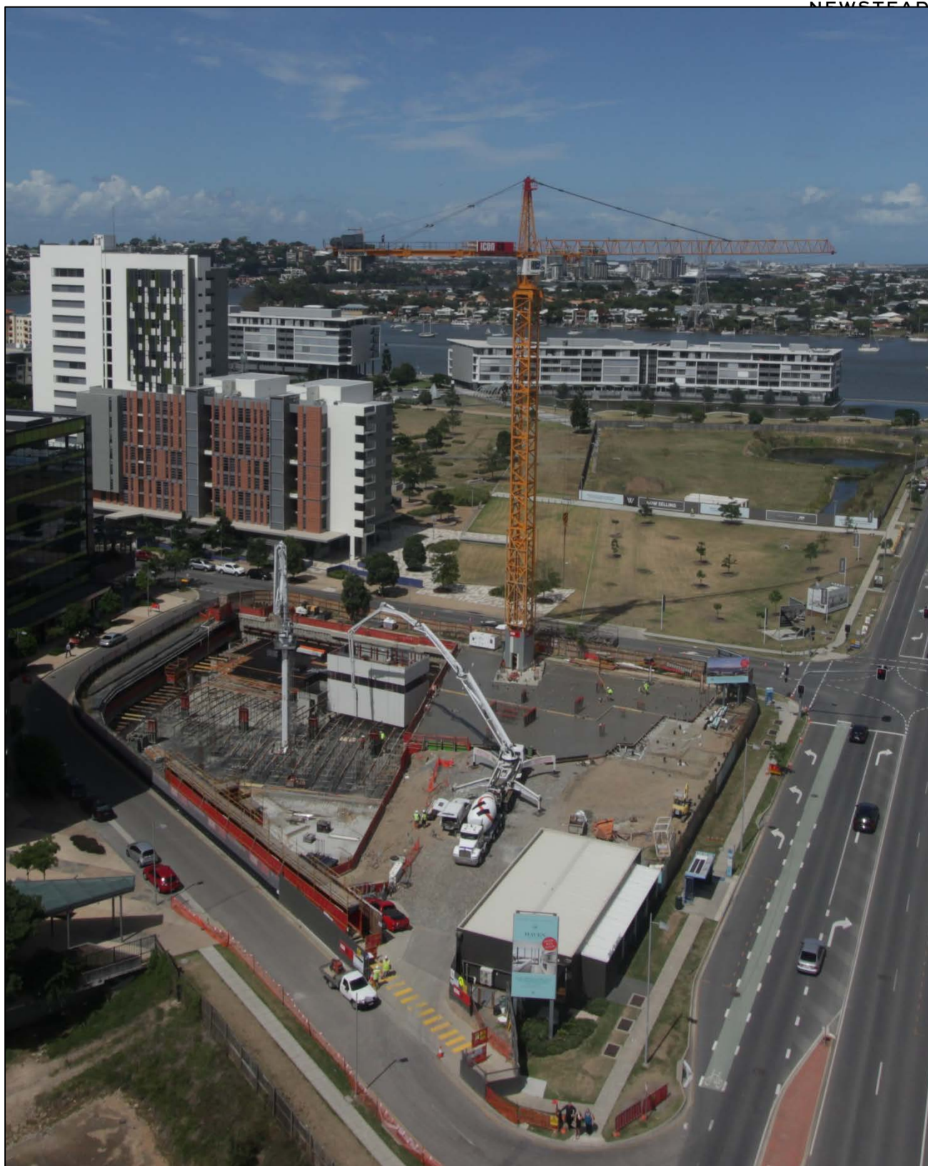
Haven Site: Construction Progress 17 th December 2015
