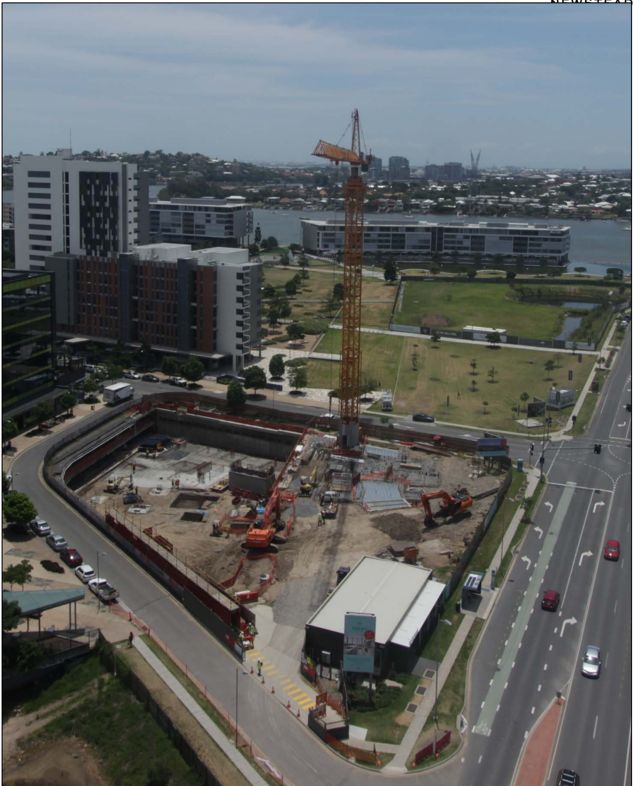
Haven Site: Construction Progress 1 st December 2015
