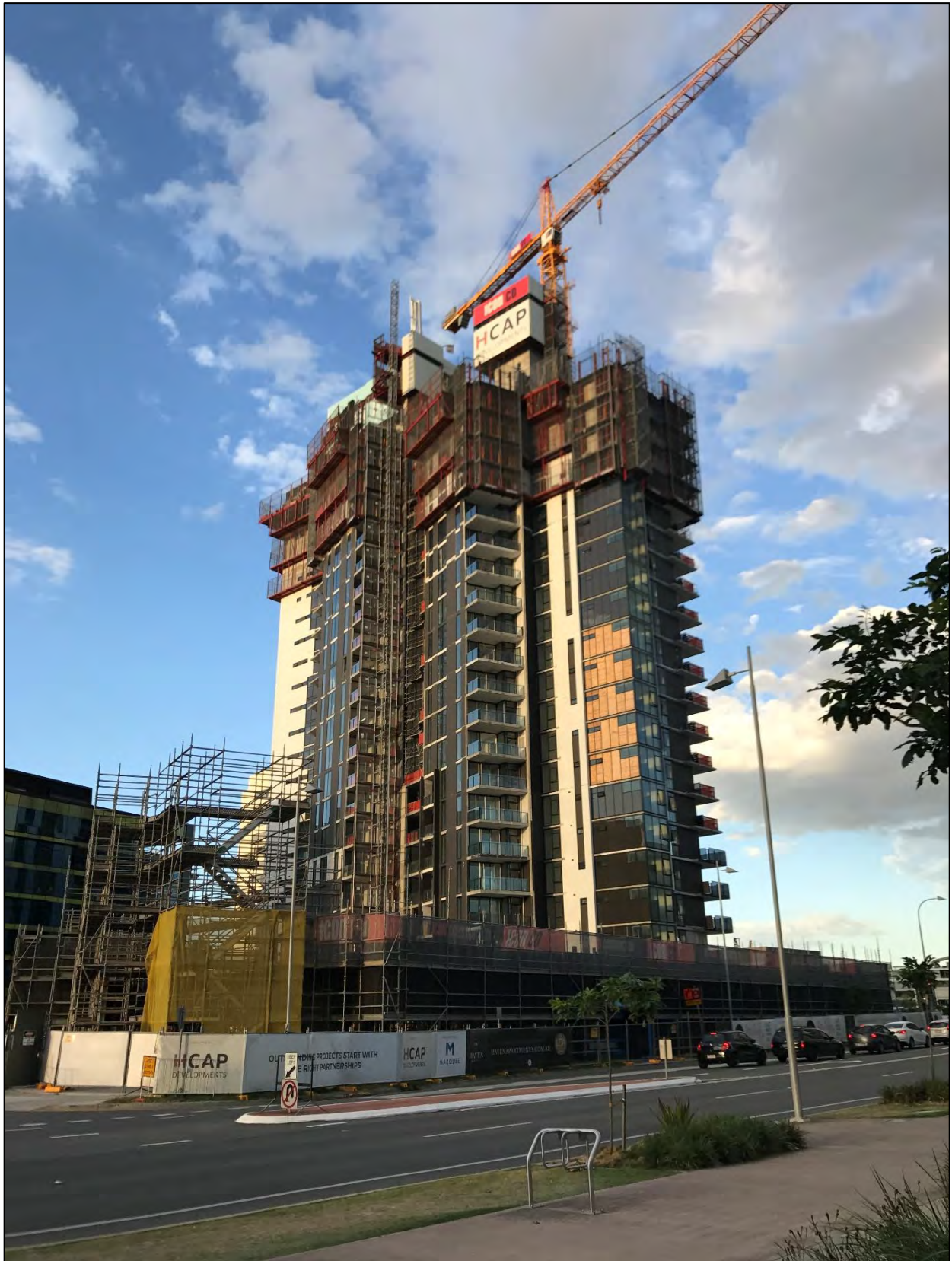
Haven Site: South West elevation with retail scaffolding along Skyring Terrace.
