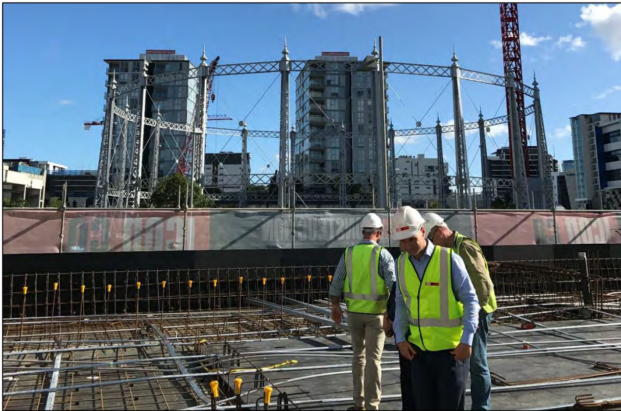
Haven Site: Project team inspecting retail mezzanine slab adjacent to Gasometre.
