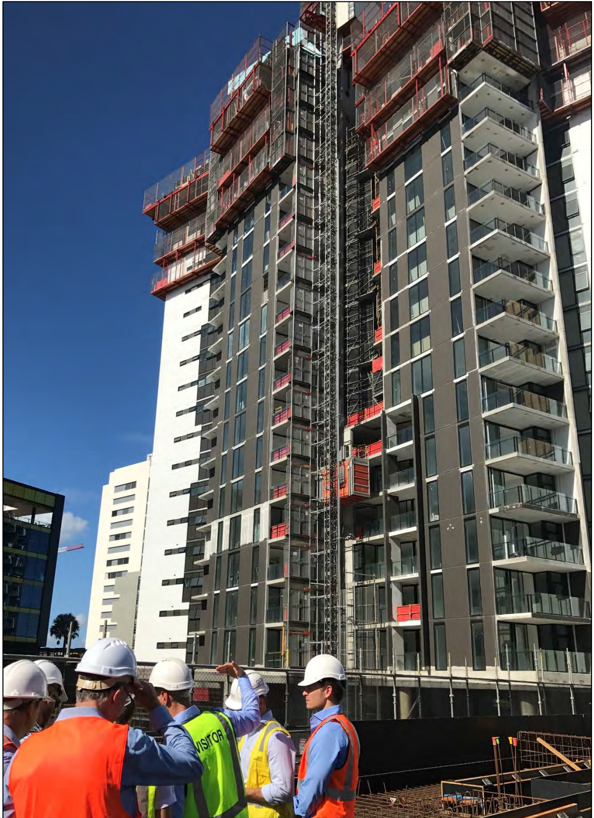
Haven Site: Project team inspecting the retail mezzanine slab.
