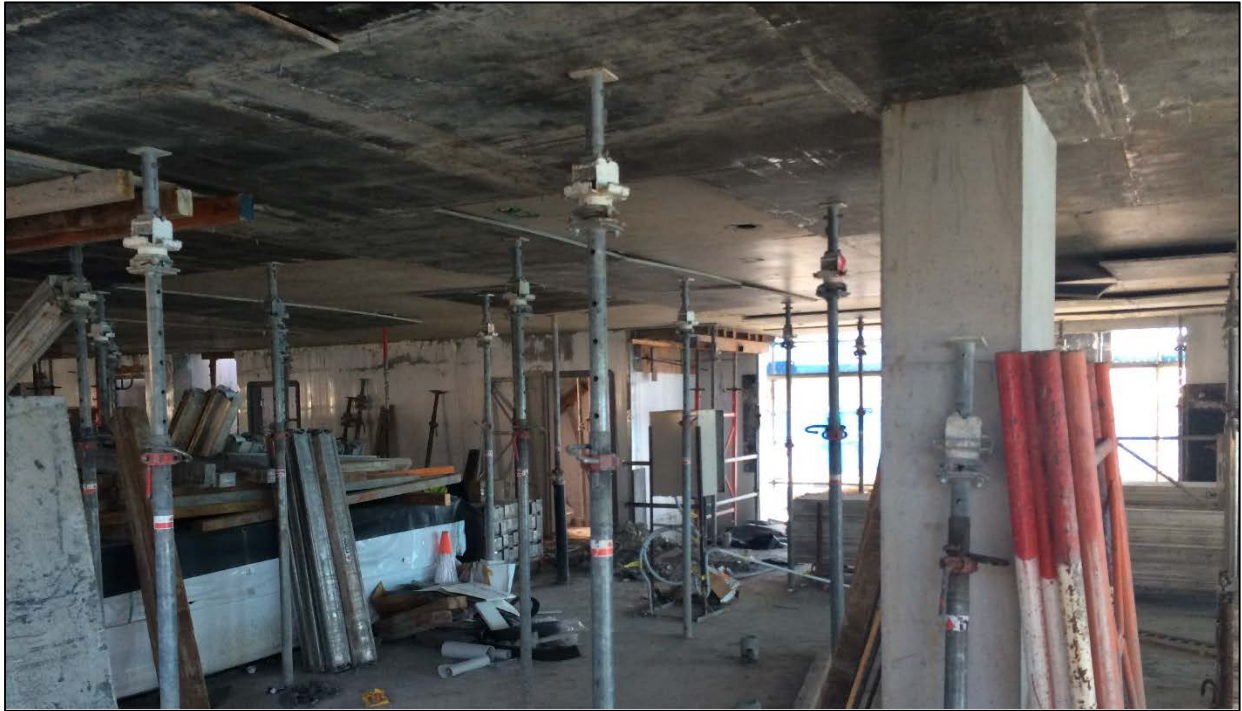
Figure 6: Level 4 – Floor slab supports remain in place while the concrete cures.
