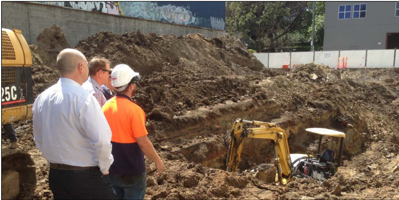
Figure 3: The bulk earthworks program commenced with excavation of site.
