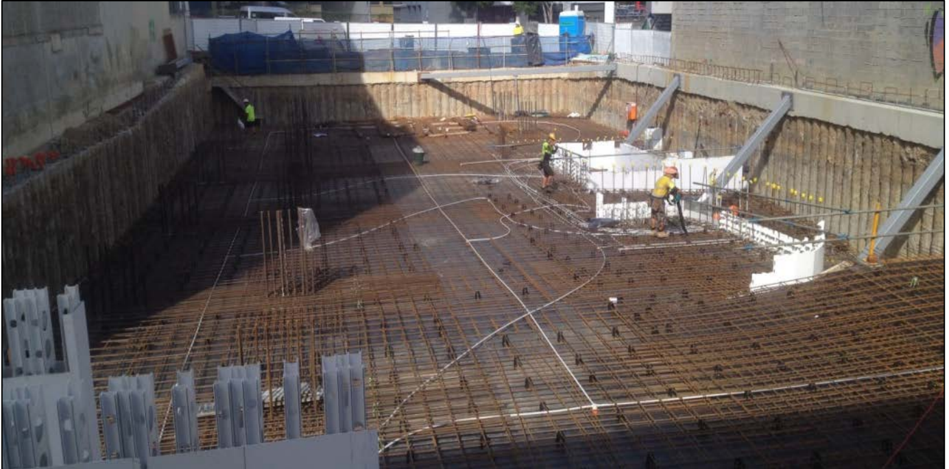
Figure 7: Reinforcing mesh is laid for the basement 1 slab.
