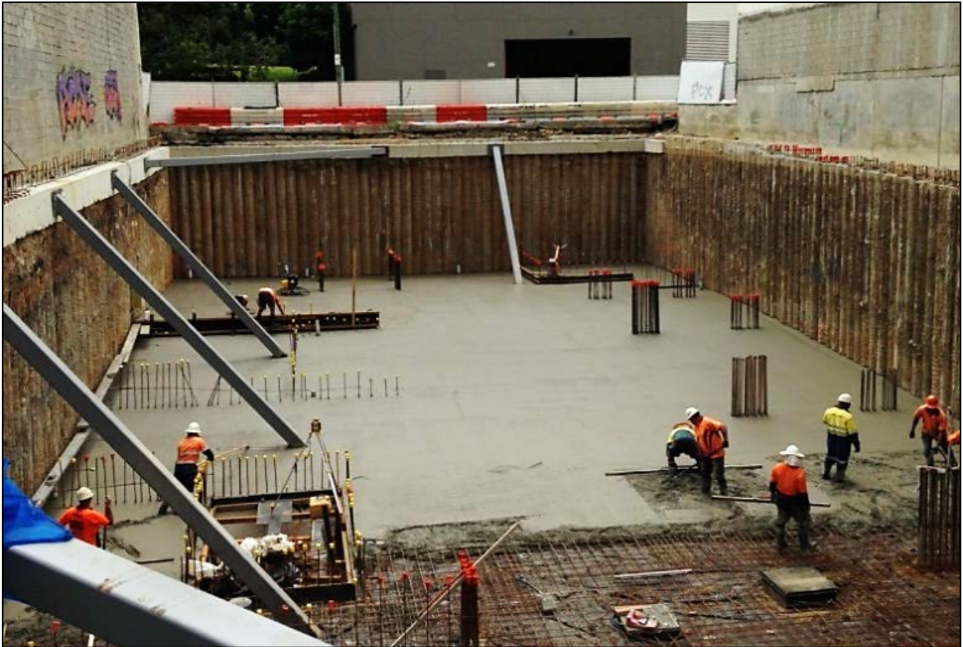
Figure 5: The basement slab is poured once the steel reinforcing is laid.
