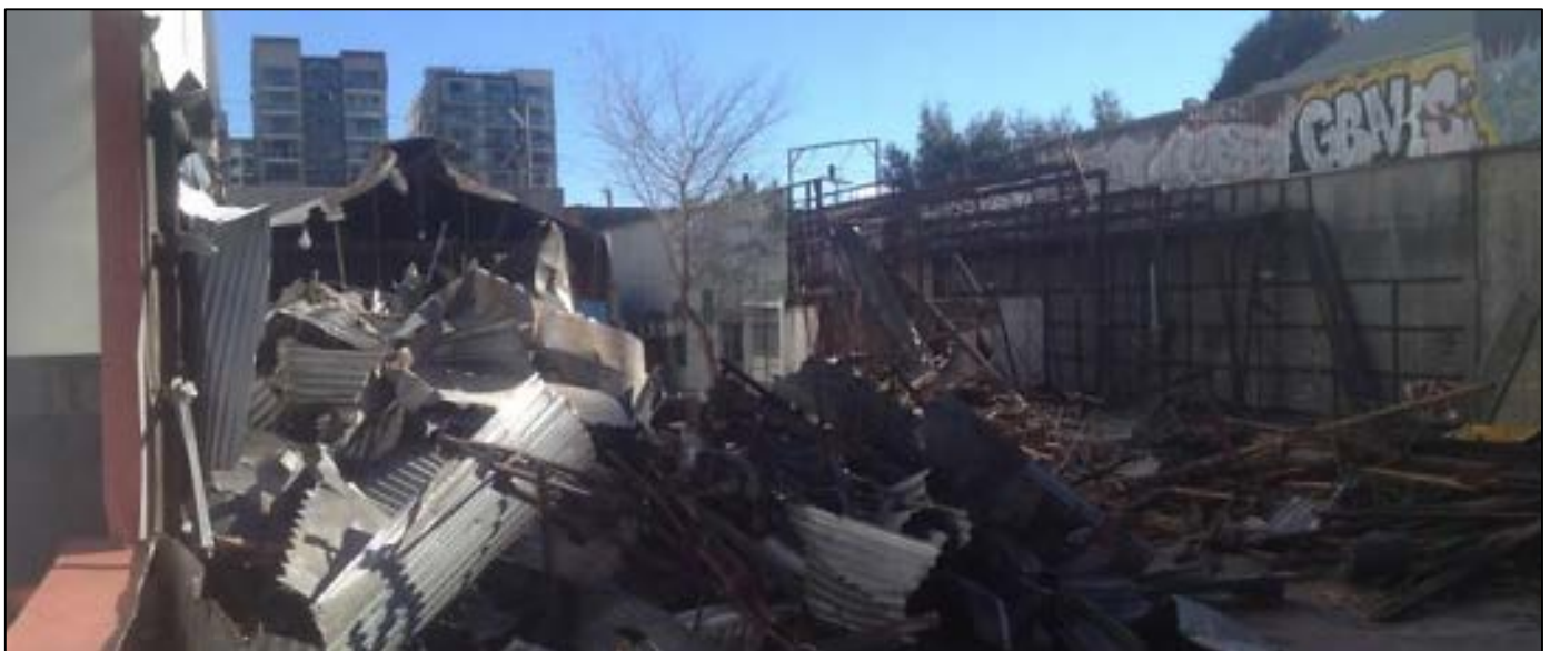
Figure 2: Existing buildings were demolished in a matter of weeks.
