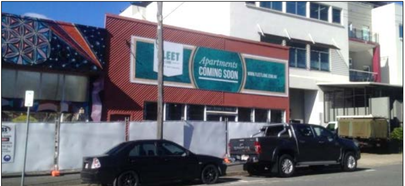
Figure 1: Demolition commenced July 2014
