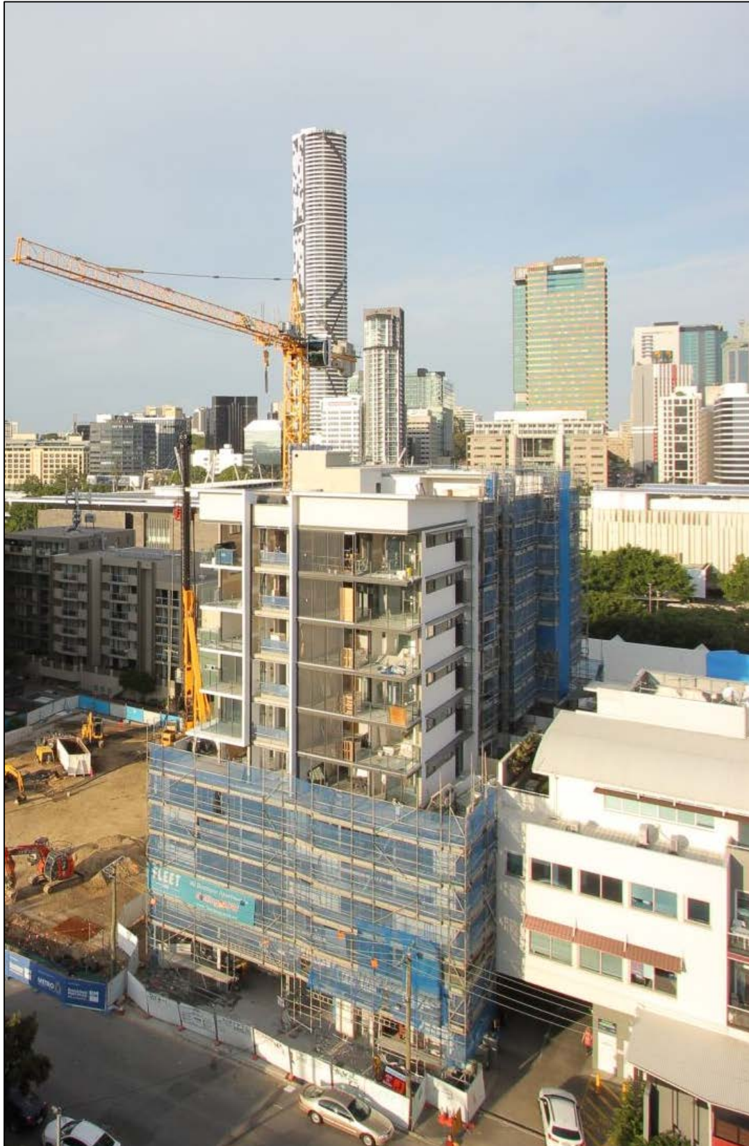
Figure 6: As scaffolding is removed, the building façade is revealed.
