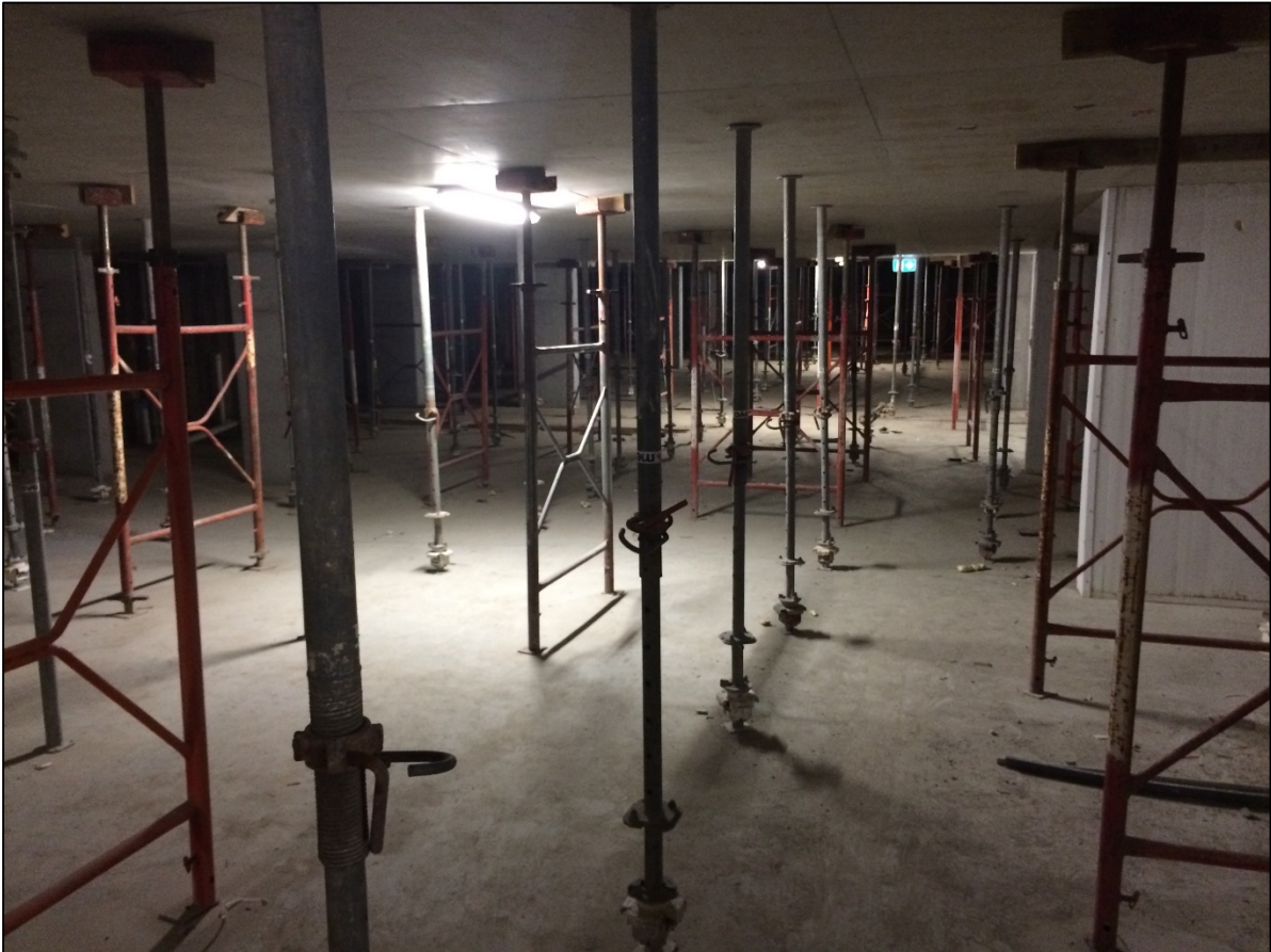
Figure 7: View of Basement 2.
