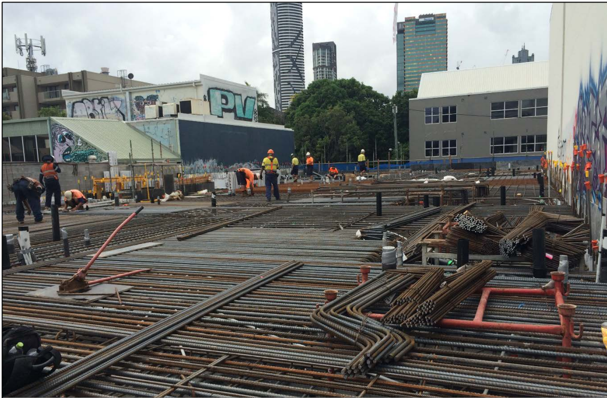
Figure 9: View of the preparations underway for the Level 2 slab pour.
