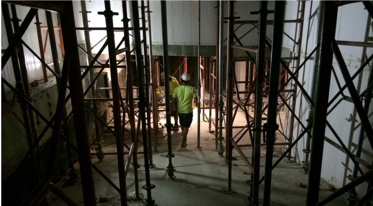
Figure 5: View down the first ramp from ground level to Basement 1.
