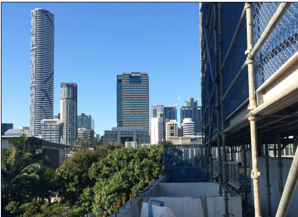
Figure 5: Level 4 view from oversized terraces.
