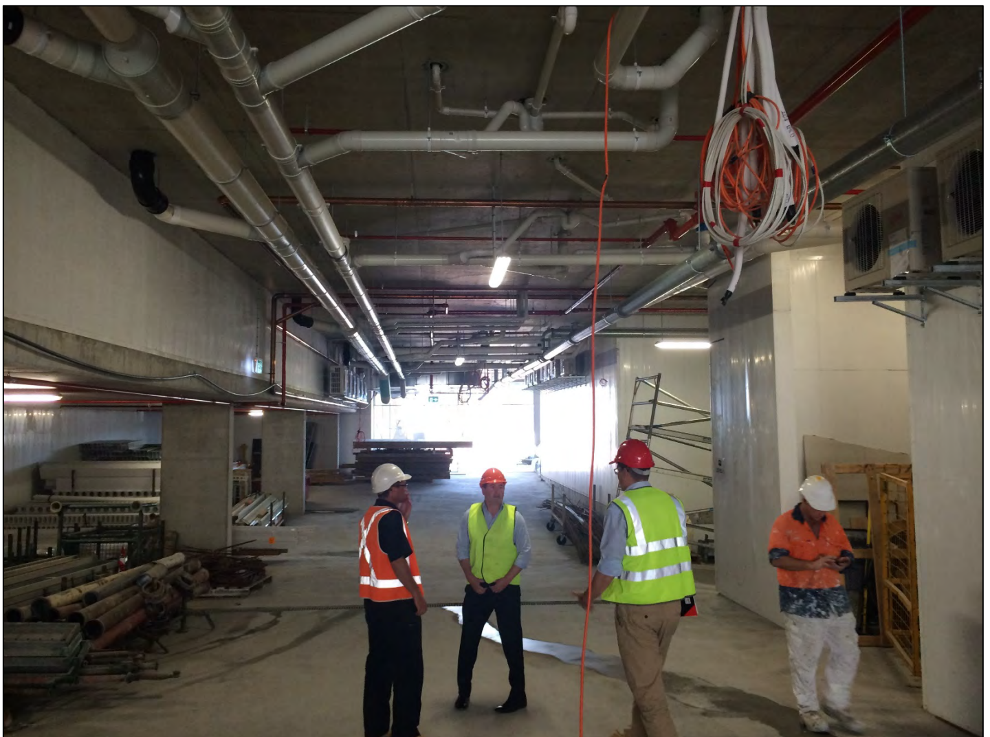
Figure 1: Ground floor driveway from Fleet Lane frontage.
