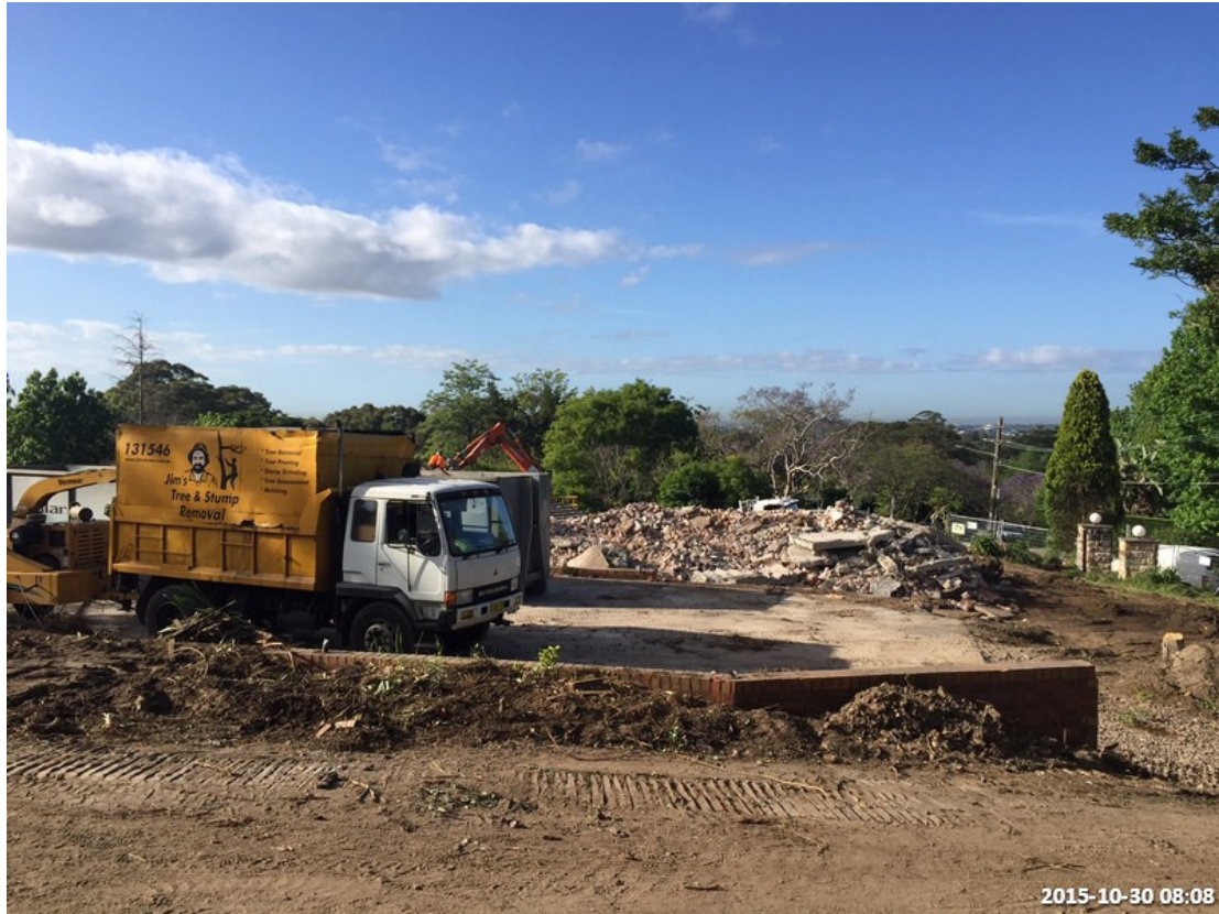
Photo 5 – The photo below shows the complete demolition of 6 Livingstone Avenue Property.
