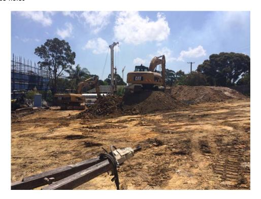
Photo 4: This photo shows the piles which have been drilled by the drilling rig. The reinforcement and concrete has been placed in the holes. These are the holes around the sewer diversion works
