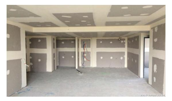
**Photo 6:** Shows the Level 1 Unit 33 (same unit 1 floor below). Initial undercoat has been applied awaiting kitchen joinery installation. Joinery works will be conducted concurrently across all levels.
