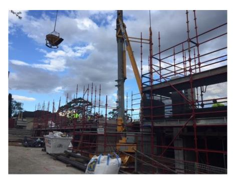
Photo 2: Shows the installation of the external scaffolding up to Level 2 West Deck. Scaffold has now been installed for the entire perimeter of the property. In the background you can also see the installation of the AFS walling system and crane.
