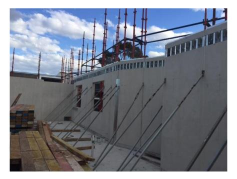
Photo 4: Shows the preparation of the Level 1 East deck prior to the concrete pour which took place on 26<sup>th</sup> May 2015. Formwork is complete, installation of steel reinforcement and services rough-ins are on-going. This photo was taken 4 days before the concrete pour commenced.
