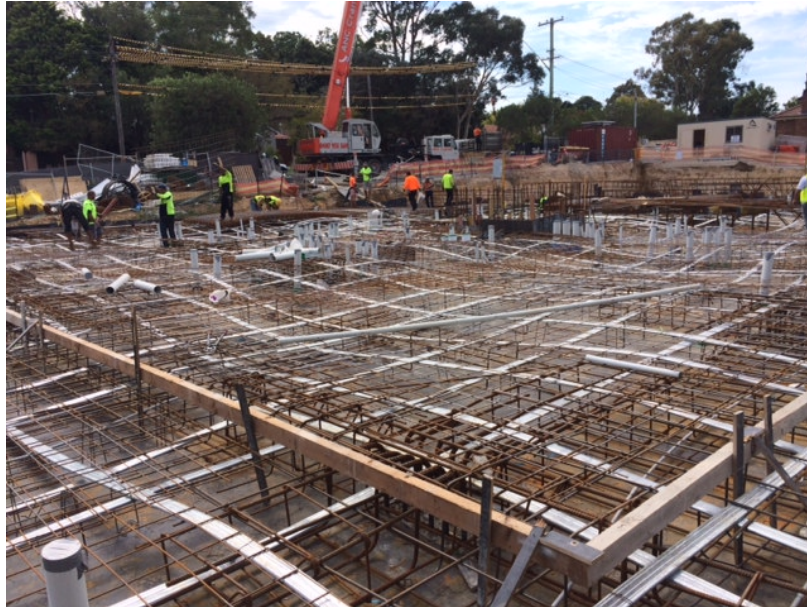
Photo 5: The last of the reinforcement mesh is being installed.
