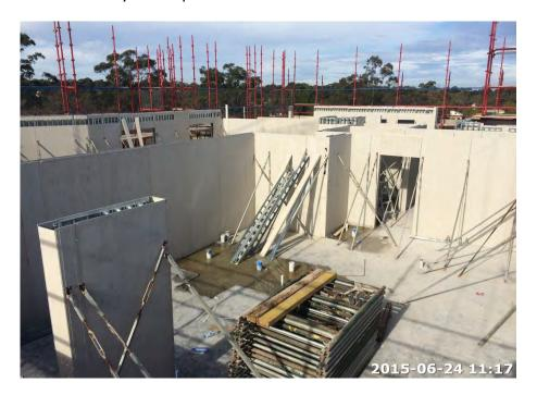
**Photo 4:** Shows that stripping of formwork and cleaning on Ground Floor West has commenced. This will free up the Ground Floor units to start receiving the finishing trades including internal studwork, sheeting and services rough-ins.
