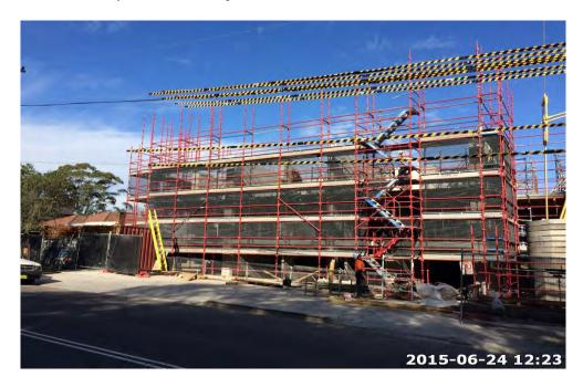
**Photo 2:** Shows the delivery of steel reinforcement (mesh) to Level 3 West Deck. All formwork and edging for the deck is completed, majority of steel reinforcement has been fixed, the AFS internal and lift shaft walls have been poured with concrete, hydraulic and electrical services installed, with the concrete pour scheduled to commence on 26/06/15.
