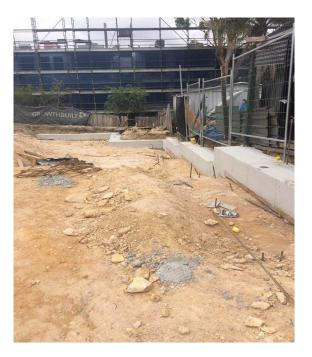
Photo 2: The sewer diversion works to the rear of the property have been excavated and the pipes have now been laid. The sewer inspection and final connection is being carried out this Friday.
