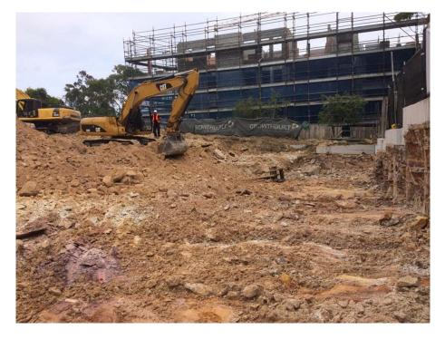
Photo 4: This photo was taken on the 19<sup>th</sup> November and shows that the first level basement has almost been excavated and removed. The bulk earthworks are approximately 40% complete. The first row of anchors has been drilled and needs to be grouted.
