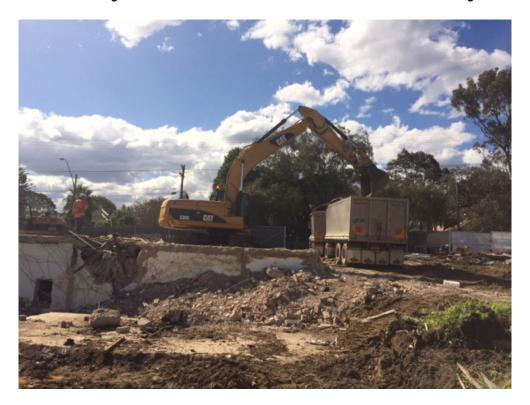
Photo 4: Demolition to No.606 has commenced as seen below. In this photo you can see the second excavator demolishing this building while the other is loading out the demolition material
