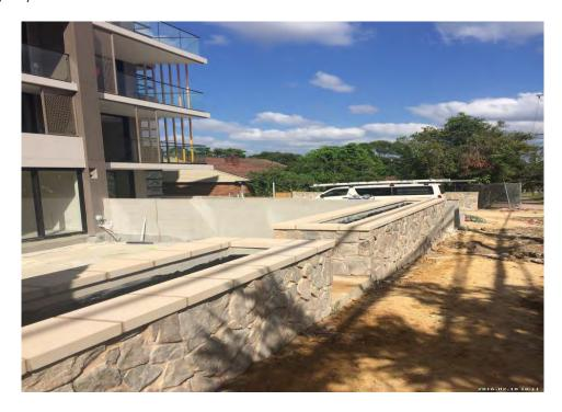
**Photo 4:** Shows the pedestrian entry into Lobby B. Also shown is the mailboxes installed into the blade wall with stone capping which will feature a structural steel glass entry awning which is currently under construction.
