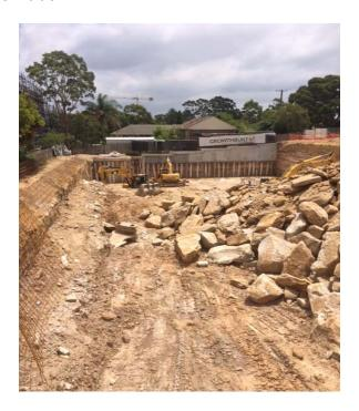
Photo 4: The bulk earthworks to the second basement on the western side has reach the maximum bulk excavation level. The plumber and detailed excavation can now commence
