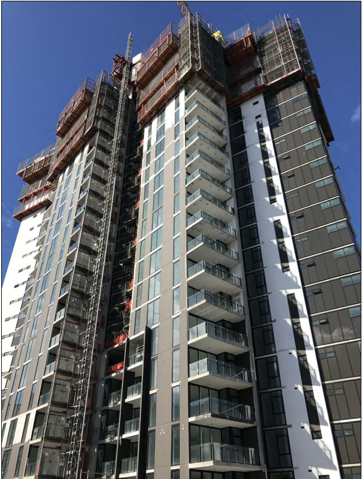
Haven Site: Western elevation.
