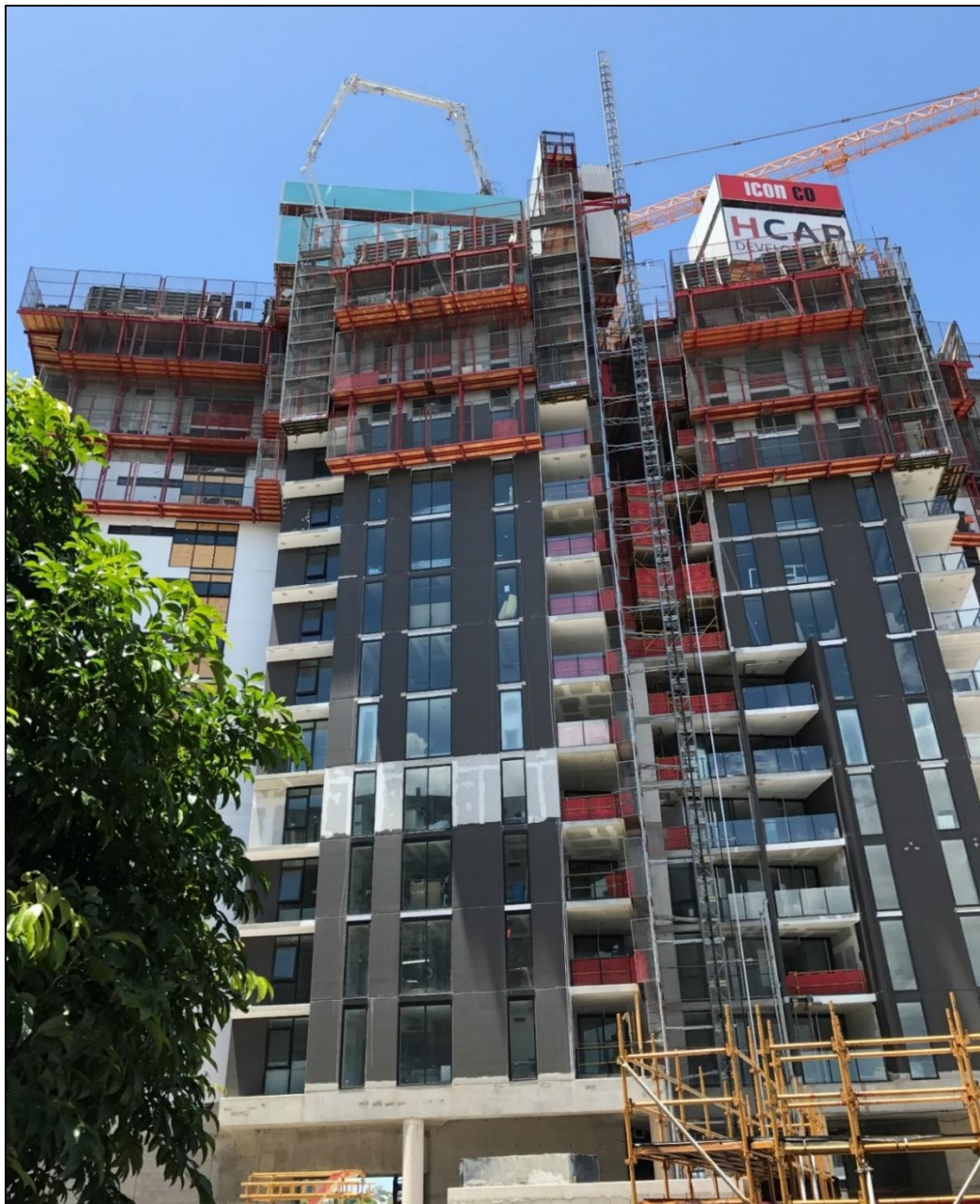
Haven Site: Western Elevation from Ground Floor.
