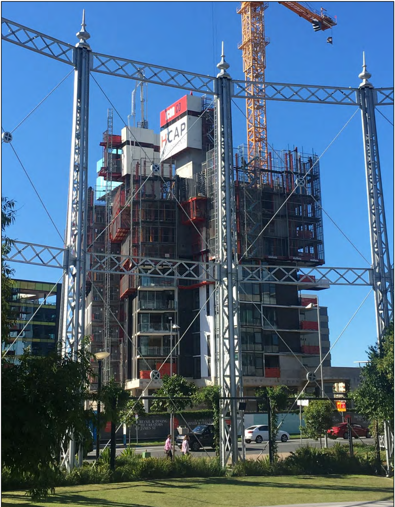
Haven Site: View of Southern elevation through the adjoining Gasworks Plaza.
