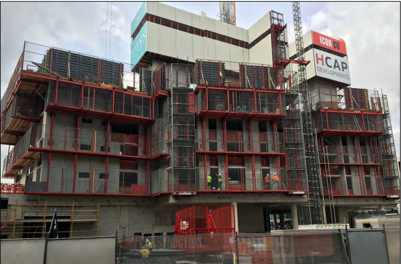
Haven Site: North Western Façade 17 th June 2016
