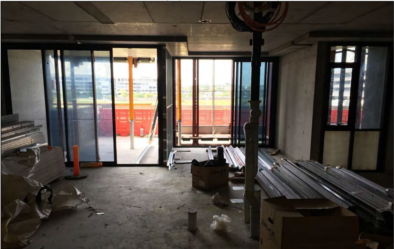
Haven Site: Installation of glazing on Level 1.
