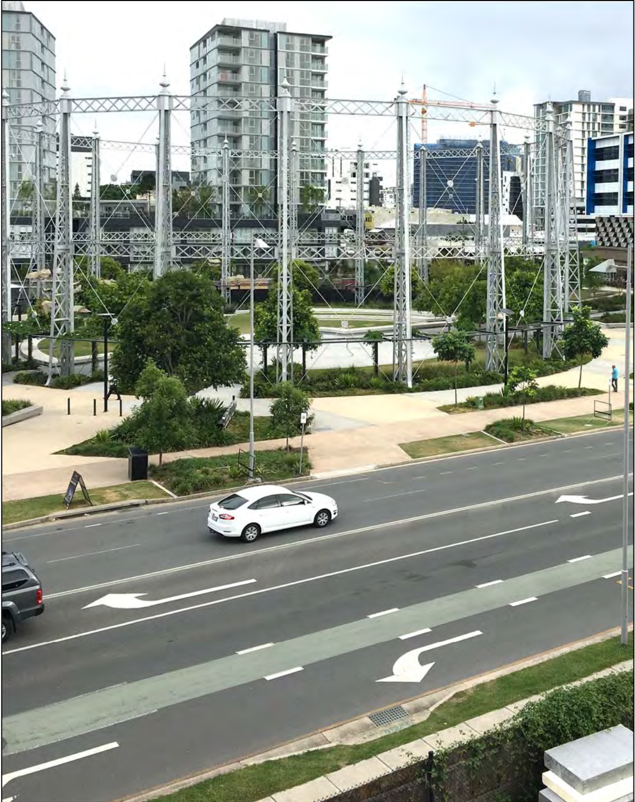
Haven Site: View towards Gasometer from Level 3 Terraces.
