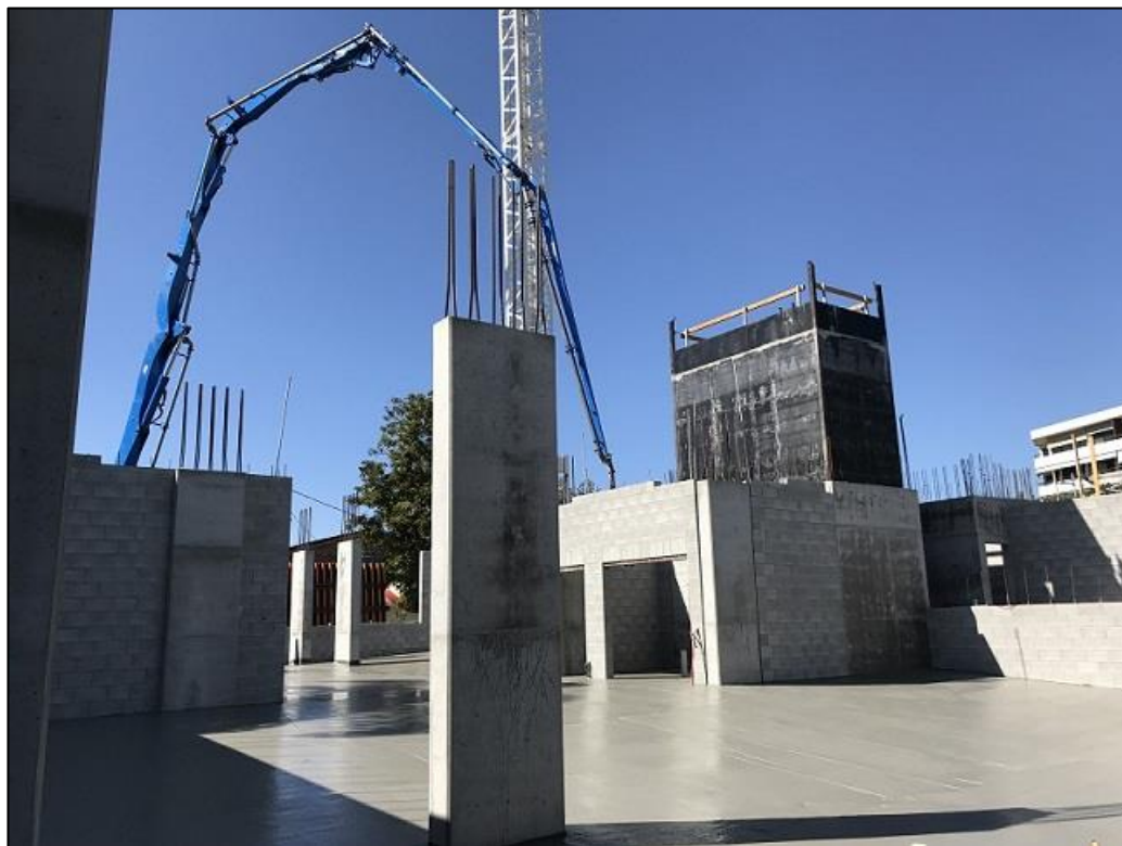
Level 1 carpark driveway freshly poured.
