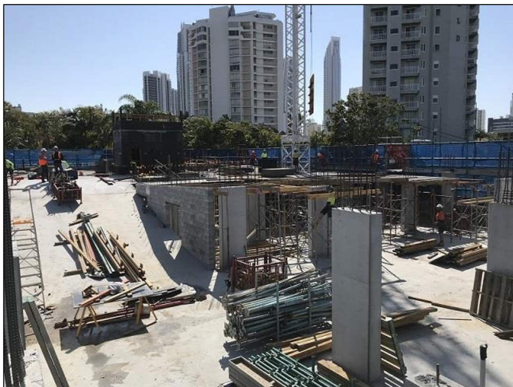
Level 2 slab formwork being installed.
