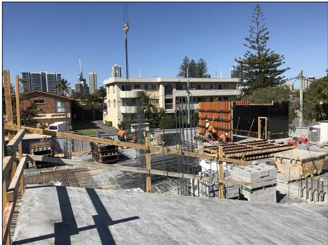
Level 1 slab and ramp to Level 2 complete.
