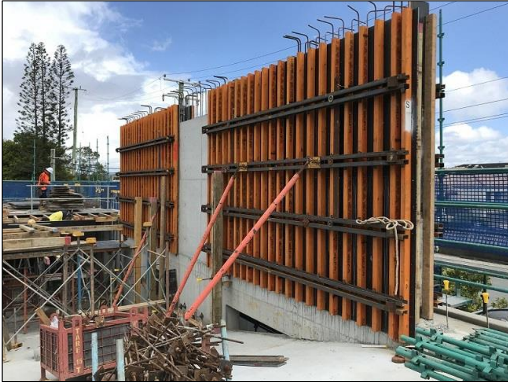
Level 2 structural walls curing.
