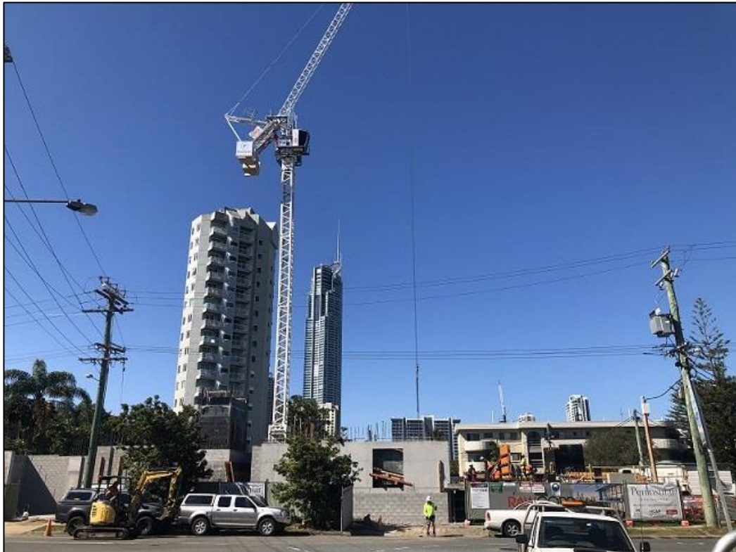
Tower crane installed with Level 1 structural work underway.
