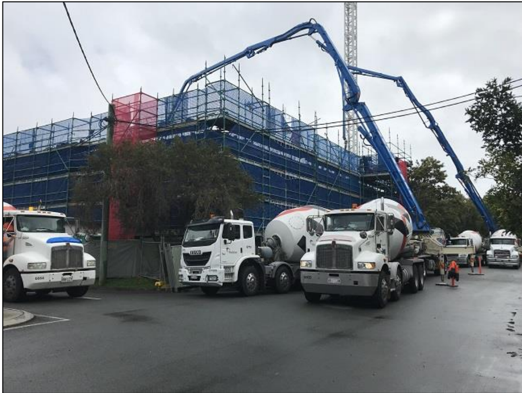
Several concrete trucks are on standby to supply the concrete pumps.
