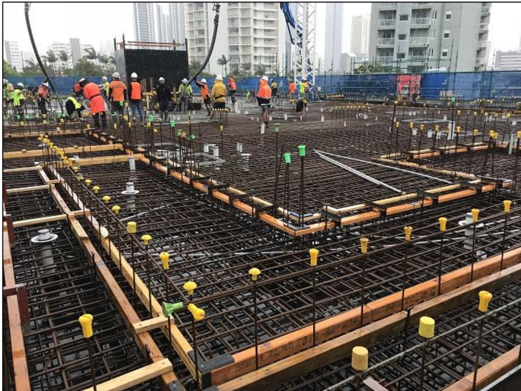
Concrete crews pouring the transfer slab.
