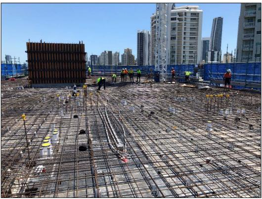
Level 4 Slab Reinforcing fixed to deck
