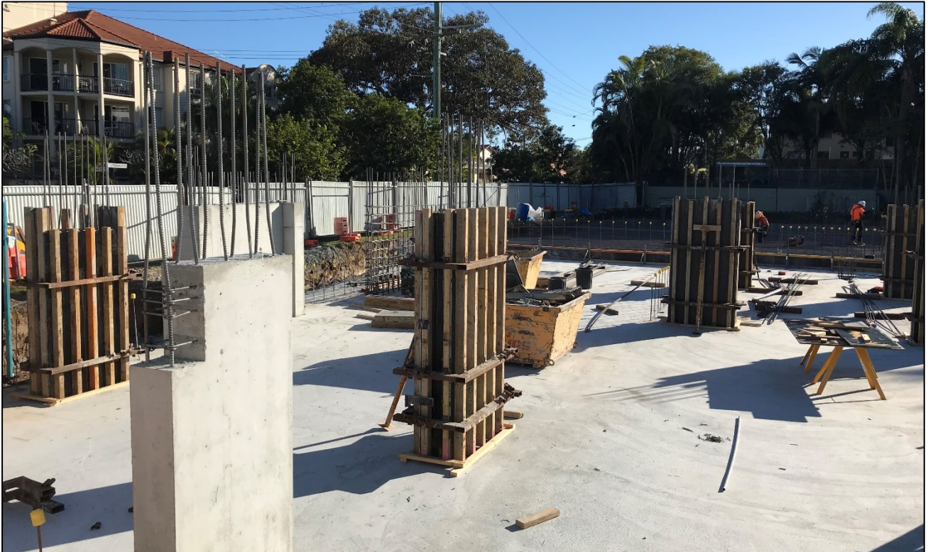
Peninsular Site: Southern raft slab with column formations.
