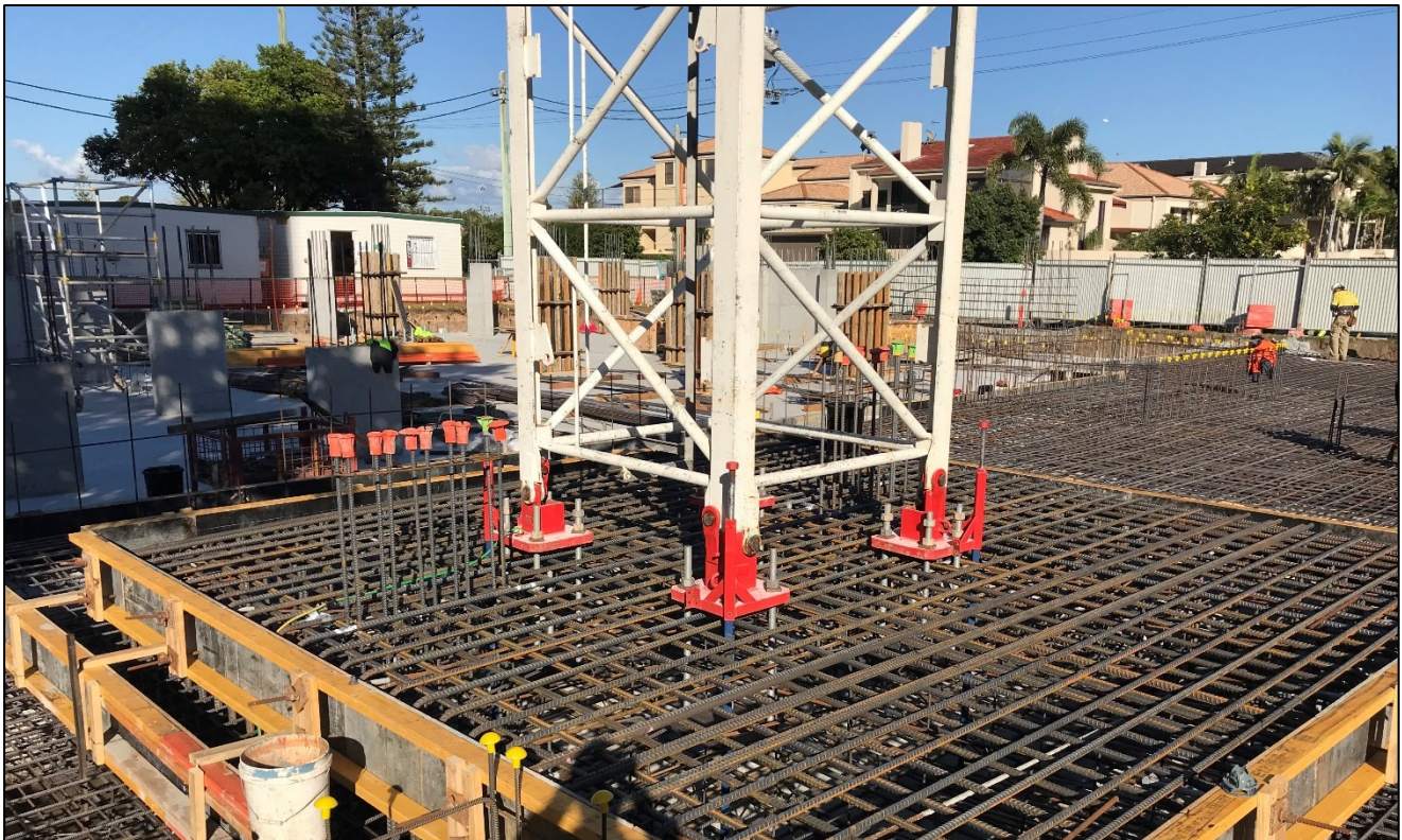
Peninsular Site: Northern raft slab and crane base steel reinforcing.
