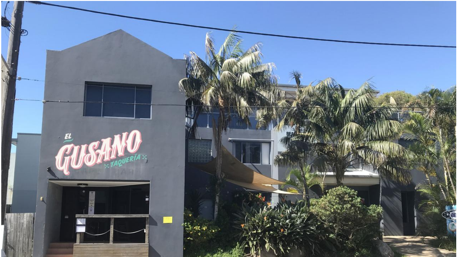
The existing building at 4 Collaroy St, Collaroy. Picture: John Morcombe
